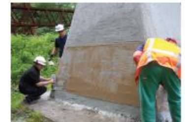
Fig. 4.1.4b—Installation of FRCCM system.
