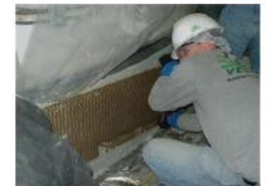
Fig. 4.1.5—Installation of reinforcement mesh on equipment base.
